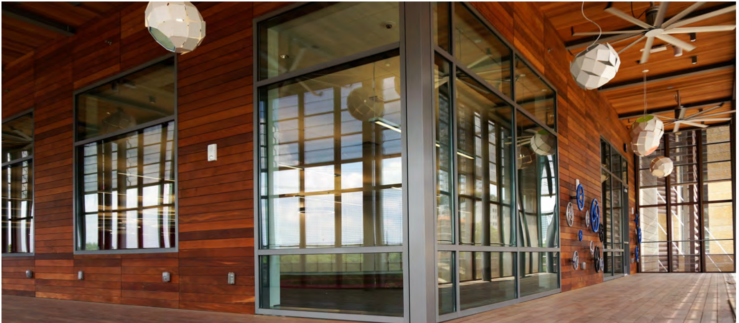
Project: Austin Central Library | Architect: Lake Flato Architect Products Used: Prime Line Western Red Cedar Vertical Grain. KD 5/4 Ipe Decking, 1 x 6 Ipe Siding with hidden cleat system---
